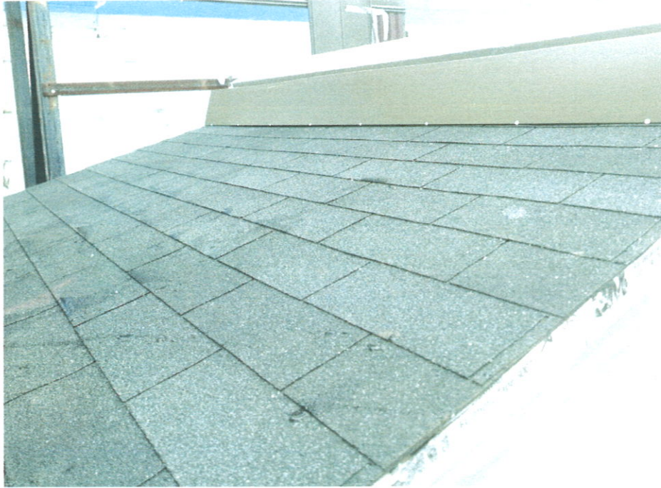
TOP OF ASSEMBLY PRIOR TO TEST
